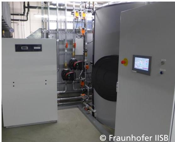
Heat pump system for heat recovery from exhaust air
